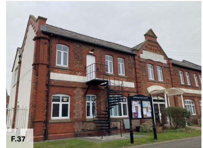
Figure 37: Rajar Building on Town Lane
