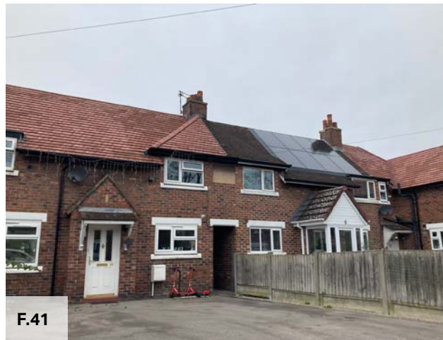
Figure 41: Housing on Bucklow Avenue
